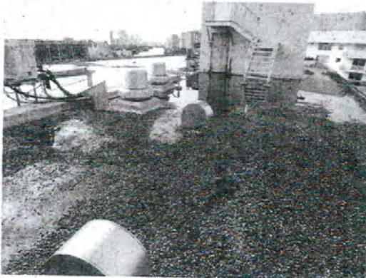
Built-Up Tar & Gravel Roof Covering
