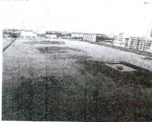
Built-Up Tar & Gravel Roof Covering
